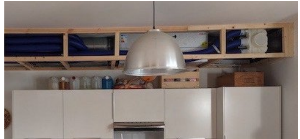
A small MVHR system in a bulkhead in a flat
