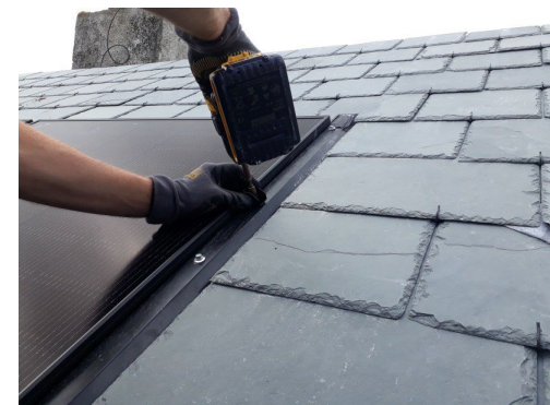
In-roof installation of solar panels in Newquay
