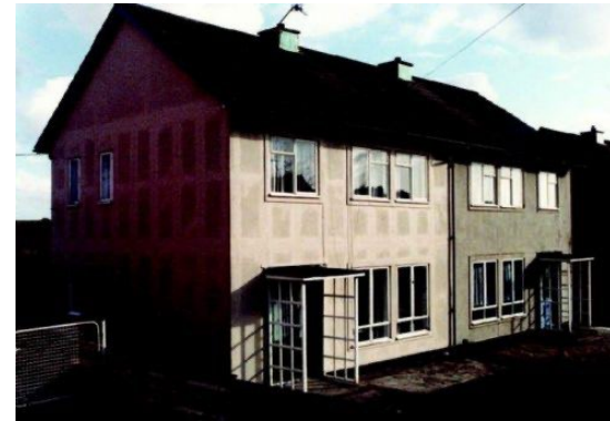
Woolaway homes. This type of construction has been classified as defective by the Secretary of state unless repaired and certified under an approved scheme (image source: Non Standard House Construction)
