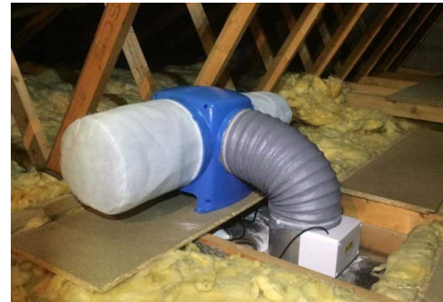
Positive input ventilation system in a loft ( dorsetelectricalsolutions.com ) and diagram showing typical set up and air flow ( precision-dampproofing.co.uk )
