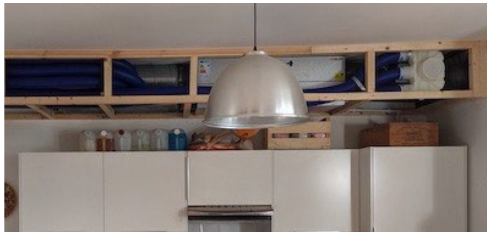
An MVHR system recovers heat from the air leaving the building and transfers it to the fresh air entering the building. This exchange heat happens without the two air streams mixing.
