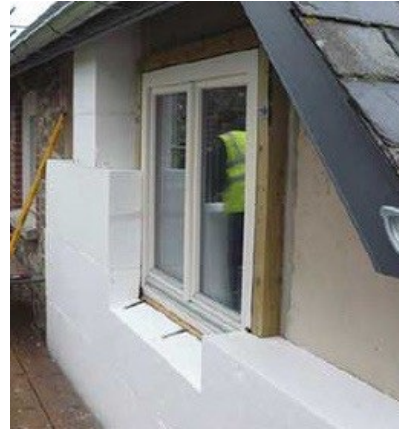
External wall insulation ( passivehouseplus.co.uk )
