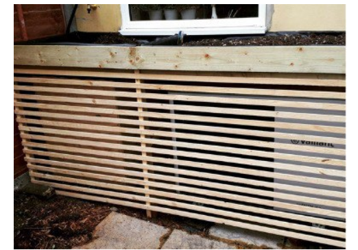
Heat pump under a window and behind enclosure
