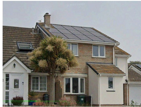
In-roof solar installation (Google)
