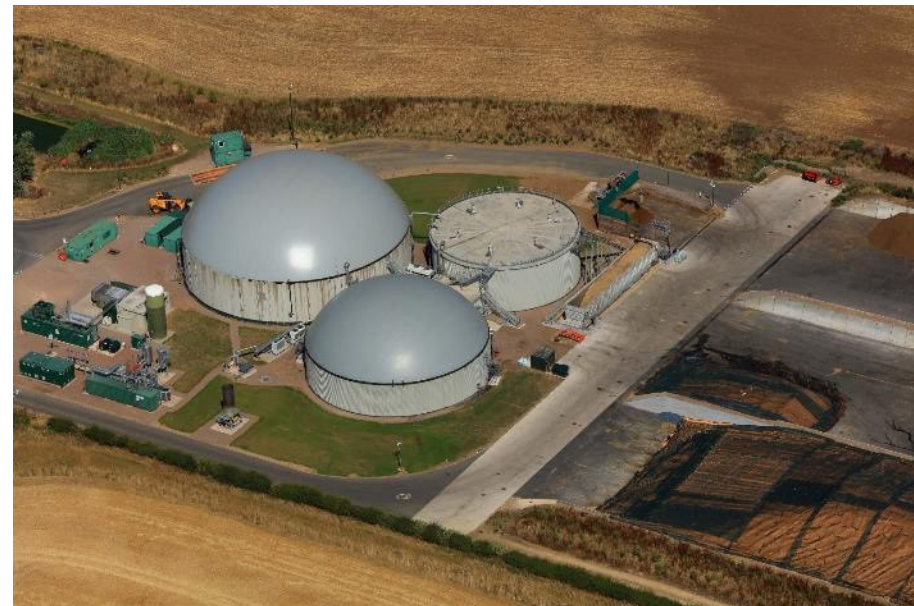
Typical anaerobic digestion facility. Biogas can be produced from waste and used to generate electricity. (image source: Renewable Energy Association)
