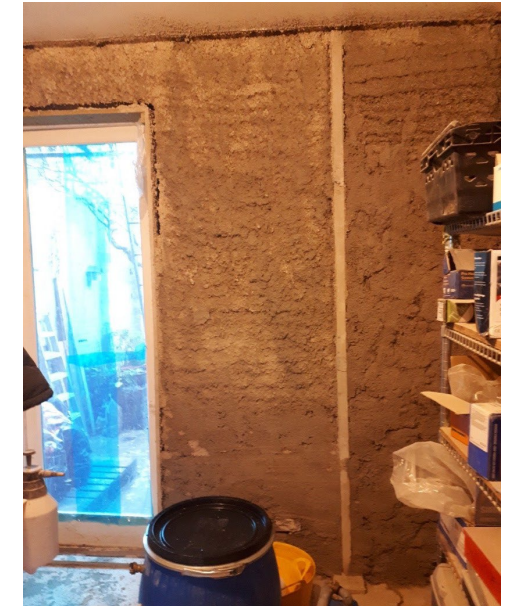
Initial coats of lime/cork plaster being sprayed onto a masonry wall (Prewett bizley Architects)
