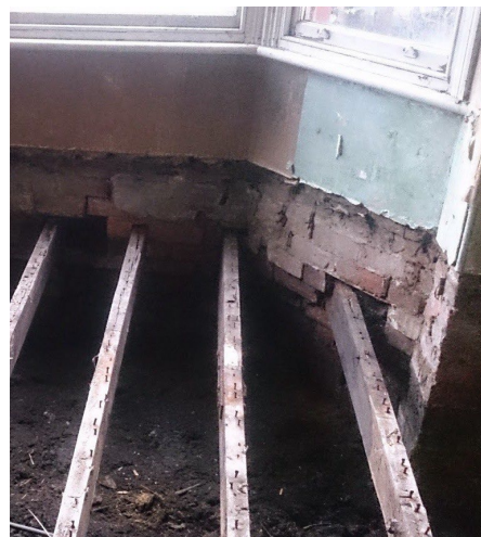
Stripping back to the structure (Image source: Eightpans) and applying airtightness tape to joist ends (Image source: Ecomerchant) will deliver best practice levels of airtightness.
