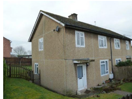
Reema hollow panel homes (image source: Non Standard House Construction)
