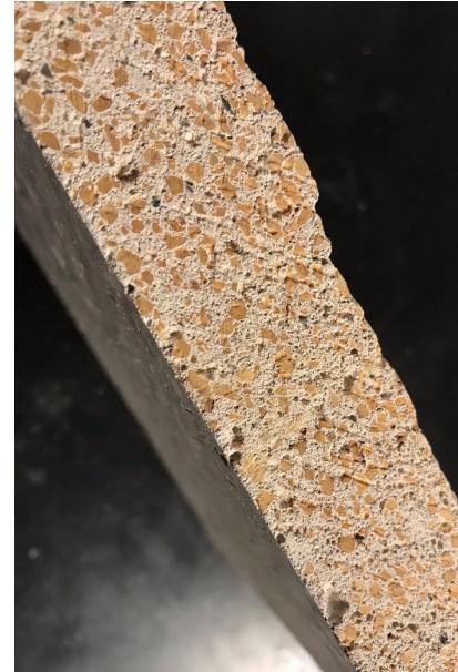
Cork granules visible in lime/cork plaster internal plaster insulation (Prewett bizley Architects)
