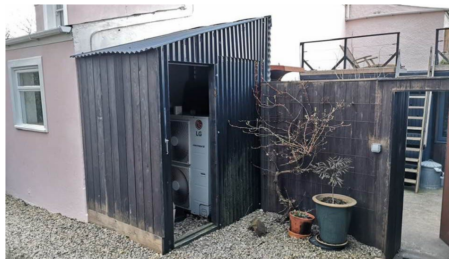
In this image, the installer appears to have lacked an understanding of a heat pump's principle of operation and has not followed basic manufacturer guidance to ensure adequate air supply. As a result the system will operate at very low efficiency, needlessly increasing operating costs (image source: Heat Pumps UK & Ireland Facebook Group)
