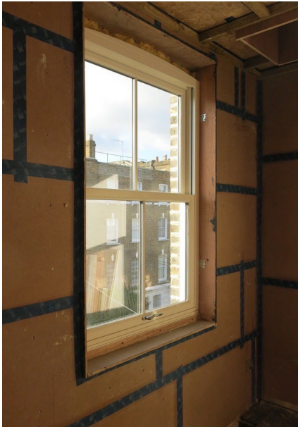
Wood fibre insulation panels fixed and taped with airtightness tape before plasterboard and batten lining (Prewett bizley Architects)
