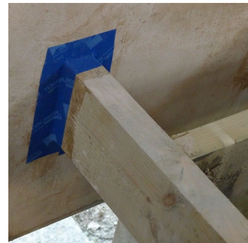
Stripping back to the structure (Image source: Eightpans) and applying airtightness tape to joist ends (Image source: Ecomerchant) will deliver best practice levels of airtightness.
