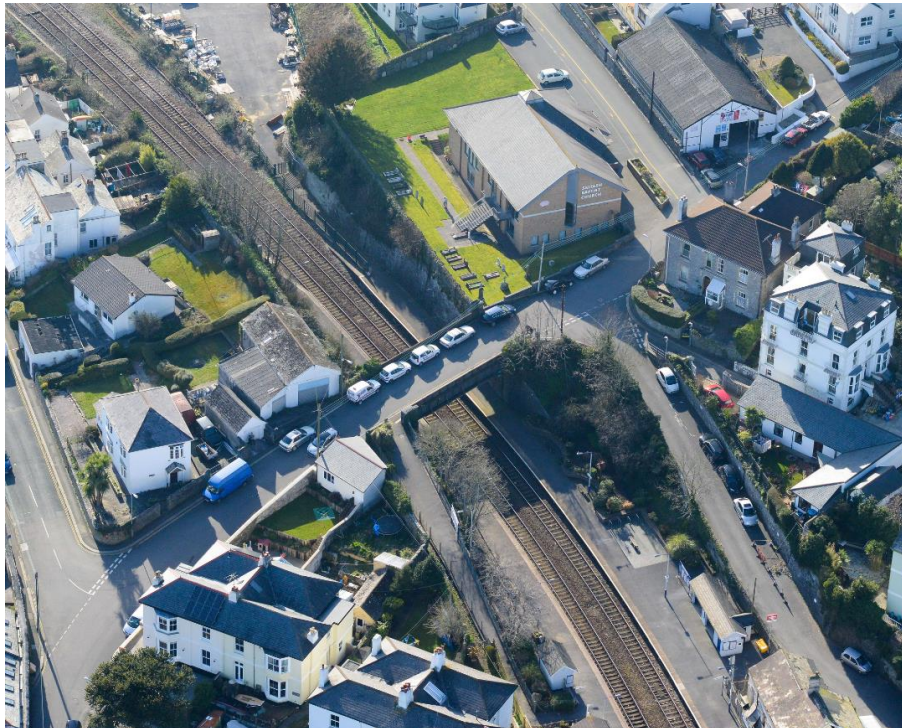
Figure E1: Platform 2 upper platform in image – with potential to extend platform to the compound area visible within top of image
