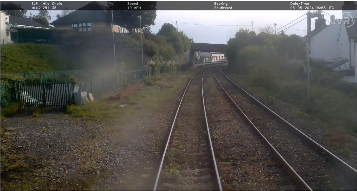
Figure 3: Overview of the site of the proposed platform extension, showing maintenance access compound and retaining wall.
