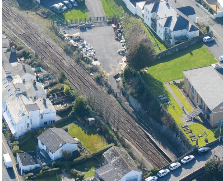
Figure 6: End of existing platform /compound area that would accommodate any platform extension – noting the compound would remain behind the platform and the RRAP maintained.
