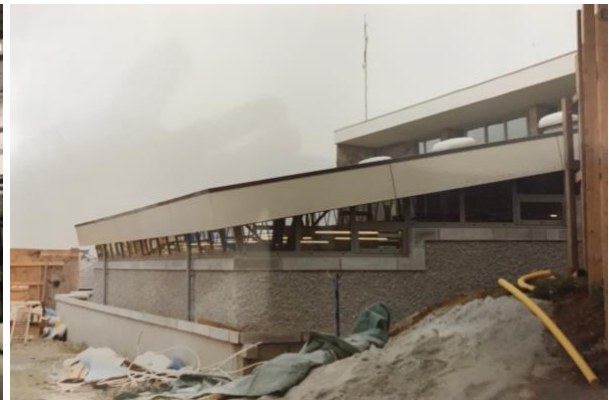
Fig 11: 1990 photograph during construction
